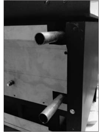
Side wetback placement with inner heat shield re-fitted
