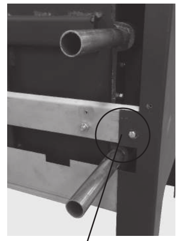
Wetback installed and side panel re-fastened. Heat shields to go back on for completion
